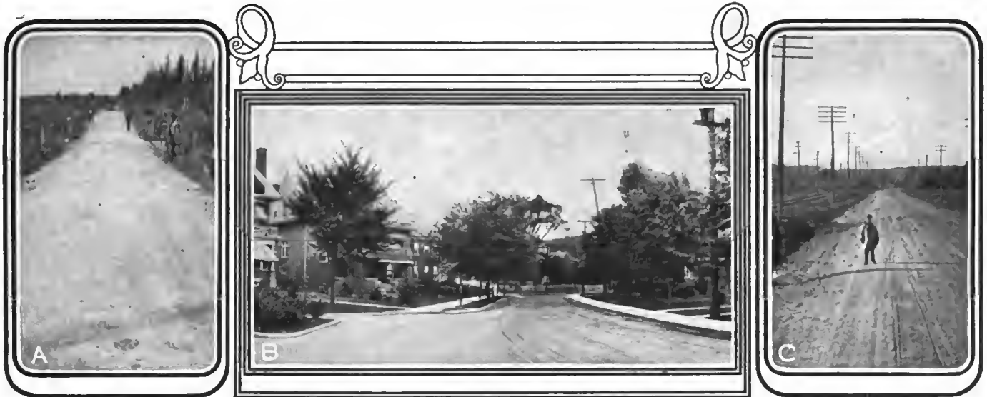
A—Building a broken-stone road through swamp in Oxford County
